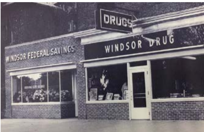
A 1950 photo of Windsor Federal Savings & Loan Association's branch office at 230 Broad Street in Windsor, CT.
