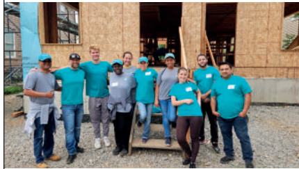
First County Bank employees rolled up their sleeves and got to work, for Habitat for Humanity of Lower Fairfield County's Build Day. Those who attended the build day, helped with tasks from framing to painting, contributing to the construction of a new house in Bridgeport. This was a fulfilling day of hard work, team spirit and community support.
