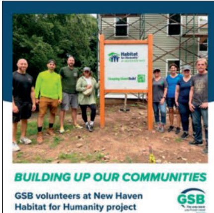
GSB volunteered to help construction efforts at the latest New Haven Habitat for Humanity project. One of our core principles is community service, because we know that when we work together, our communities thrive.
